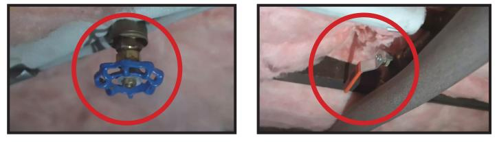
Locate the shut-off valve for the water line that enters your house. Don't try to turn off the street valve at the cement box at the curb, this valve is extremely difficult to turn and requires a special tool. Make sure that the valve can be completely shut off. Your valve may be rusted open, or it may only partially close. Make repairs before the day of the disaster. Label the valve with a tag for easy identification and make sure all staff know where the valve is located.
