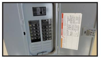
There may be times when you need to turn off the electricity to your building, for example prior to expected flooding. It is wise to teach all staff members where and how to shut off the electricity, and to properly label of your breakers.
